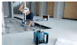
Convenient leveling of floors, concrete and all interior and exterior surfaces
